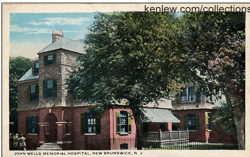
Figure 3.1. John Wells Memorial Hospital New Brunswick, New Jersey. Source: Kenlew Collection, “New Brunswick,” http://kenlew.com/collections .
